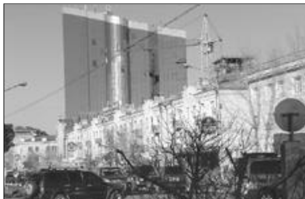
The Mongolian Development Research Center in central Ulaanbaatar, surrounded by banks, and other financial institutions.
