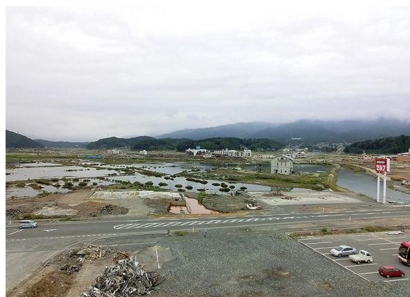
Continuous flooding in the city of Rikuzentakata associated with ground subsidence following the earthquake
