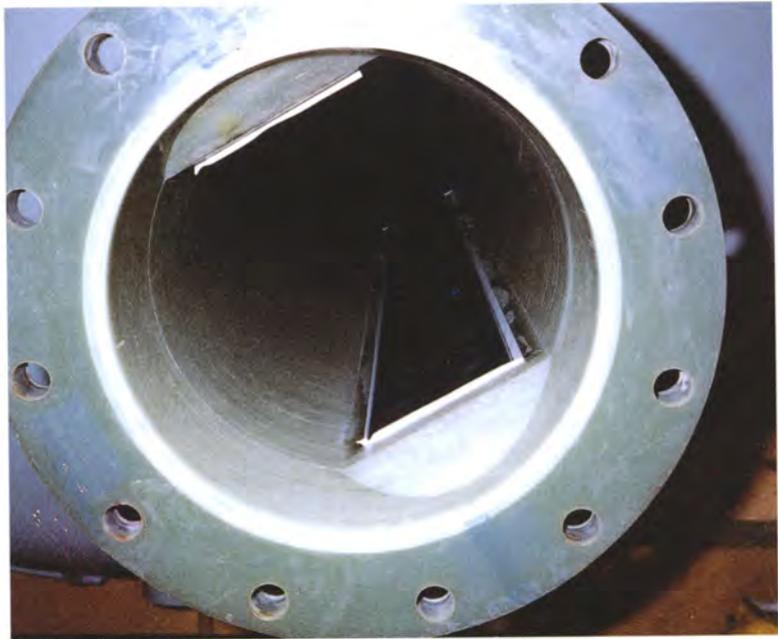
Photo 7.2 Electrodes seen from the end of a seawater duct.
