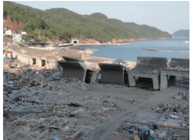
Figure 5-3-2 Damage to the coastal levee and the residential area (Touni, Kamaishi City, Iwate Prefecture)
