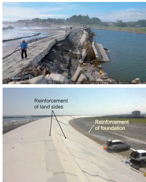
Figure 5-3-3 Top : Typical break of the coastal levee (Soma City, Fukushima Prefecture) Bottom : Restored coastal levee(Watari Town, Miyagi Prefecture)
