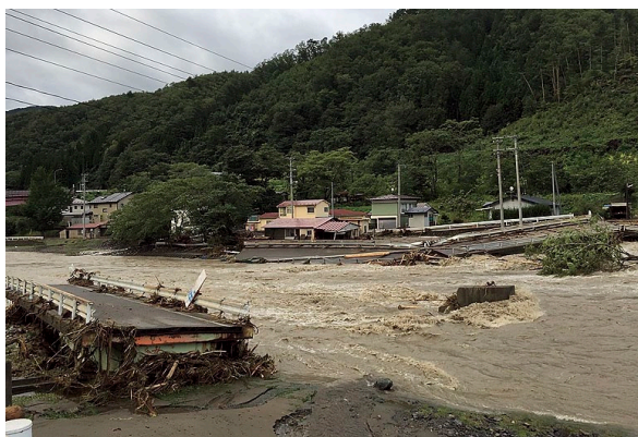
The Hikage Bridge in the Moichi district of Miyako City was washed away during floods caused by Typhoon Lionrock.
