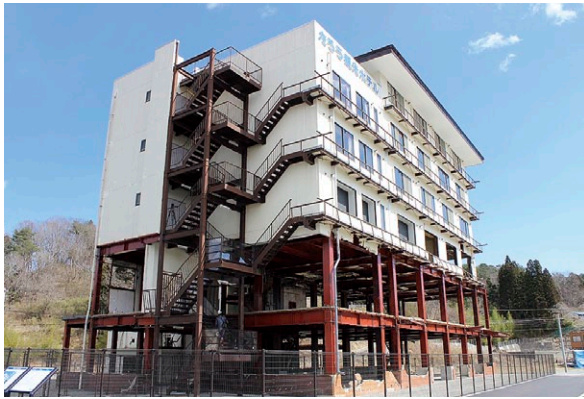
The first “earthquake disaster ruin” in Japan, the former Taro Kanko Hotel. This is an important facility for Learning Disaster Prevention.
