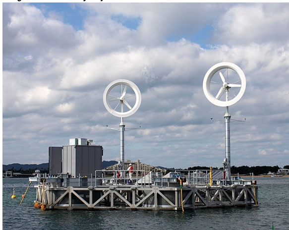
An energy farm totaling 8kW, comprising an 18m-diameter floating platform, two 3kW lens wind turbines and a 2kW solar panel, installed on December 4th, 2011.
