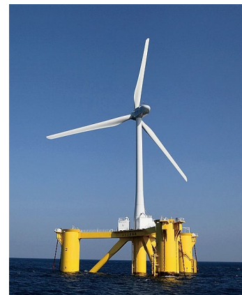
2MW downwind floating offshore wind power facility (Photo source: Fukushima Offshore Wind Consortium)
