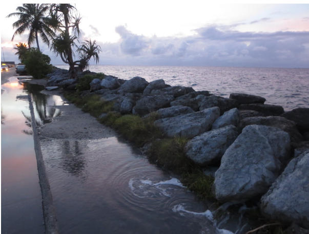
Photo 1: Seawater flowing ashore through gaps in a levee during high tide (Majuro, RMI)
