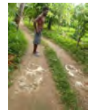
Improvement of village path
