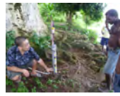
Water Level Gauge and Warning System operated by the community
