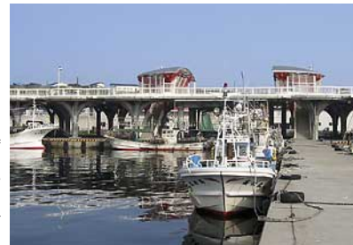
Man-made ground constructed at the port of Okushiri Island (The man-made ground can be used for parking and events activity in ordinary day as well as for evacuation from tsunamis.)
