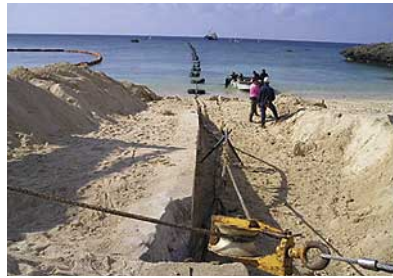
Cable landing in Miyako for submarine cables running to and from Okinawa-Honto Island and Miyako Island
