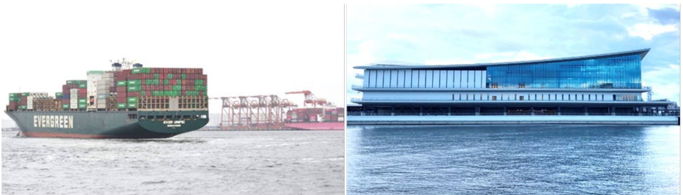
Figure 10. Port of Tokyo and its International Cruise Terminal
