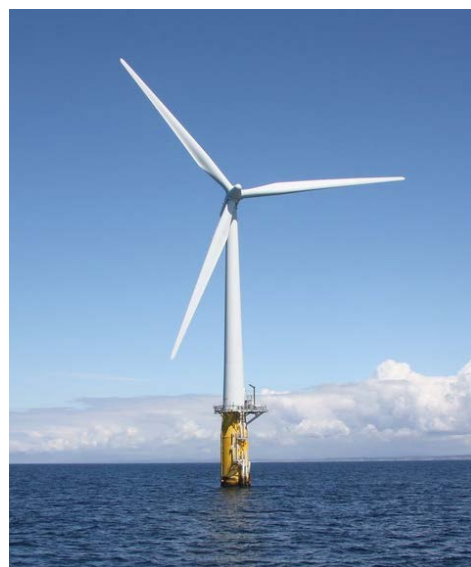
Figure 2: Floating offshore wind power at Hywind Scotland
