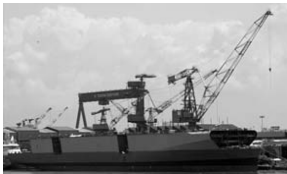
The Indigenous Aircraft Carrier (IAC) being constructed at the Cochin Shipyard
