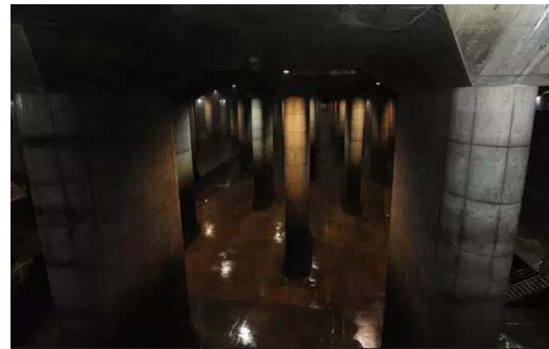
Excellent drainage system in Jasper county, Japan (日本埼玉县) (Photos from Internet, 2019)
