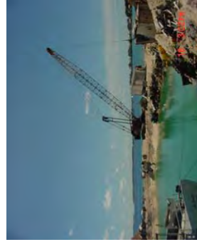
Hydraulic dragline dredging of coastal area
