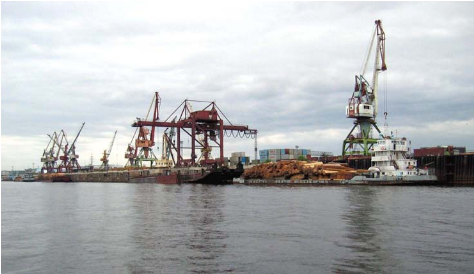
Figure 4 Cargo Handling Facilities on the Lena River
