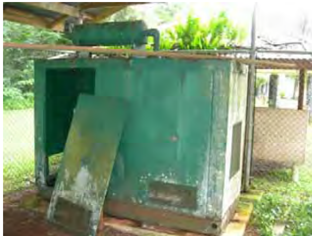
Figure-4 Emergency Diesel Engine Generator (DEG) in FSM
