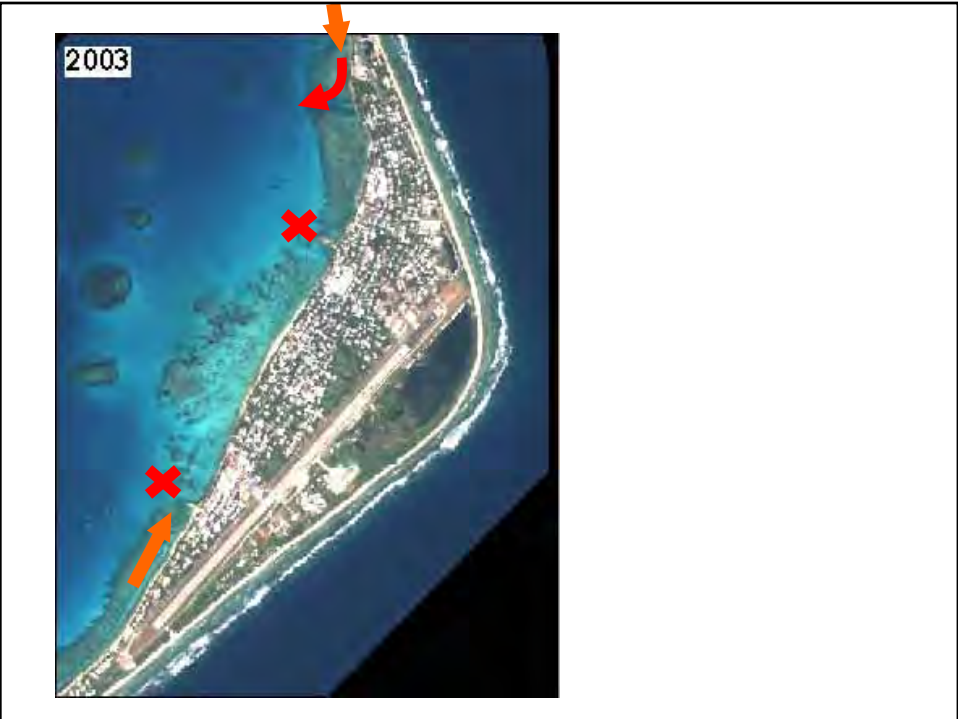
Figure 8. Sand transportation along the lagoon-side coast is blocked by the jetties and leaked through the dredged boat channels.
