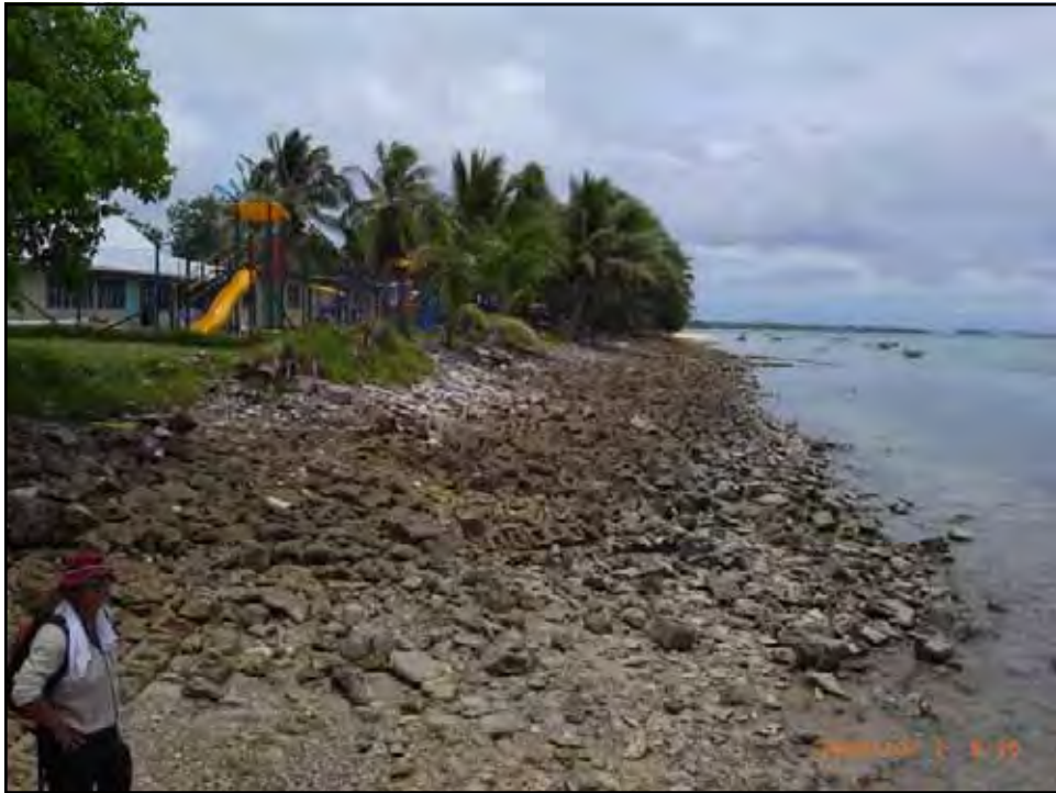
Figure 9. Collapsed seawalls.
