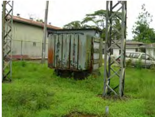
Figure-5 Substation Transformer in FSM
