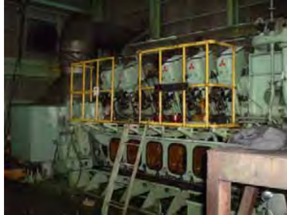
Figure-3 Diesel Engine Generator (DEG) in Palau
