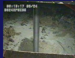
Drilling into 308°C hydrothermal reservoir at Suiyo Seamount, Izu Arc (Archean Park Project, Japan)
