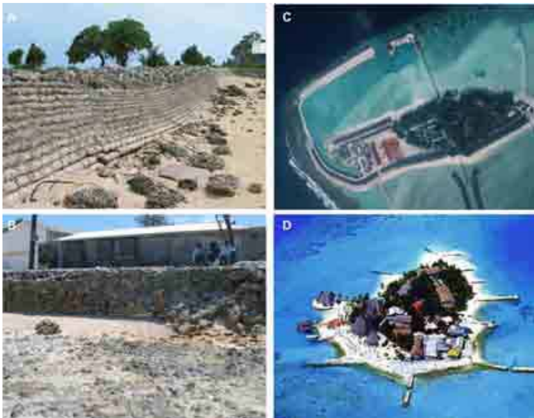
Figure 1. Examples of typical engineering structures and anthropogenic modifications of shorelines in small islands. A) Sand bag seawall in Tarawa, Kiribati. B) Vertical coral block wall in Majuro, Marshall Islands. C) Boat harbour development and breakwater design in the Maldives. D) Use of groynes to stabilise a small island in the Maldives.
